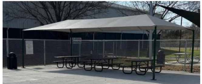
Example of 15' x 30' hip-roof shade structure
